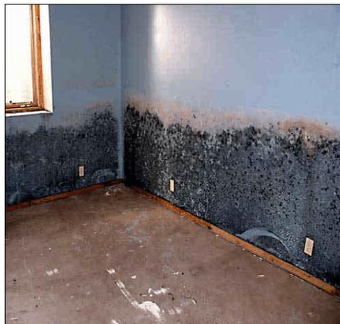
mold growth) should be removed and discarded. Wallboard should be cleaned or removed at least six inches beyond wet or water-damaged areas or visible mold growth (including in hidden areas in wall cavities).
