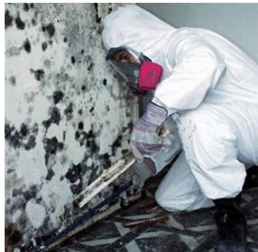
Furnishings should be removed from the area. Ventilation ducts and grills, other openings, and remaining fixtures or furnishings should be covered with plastic sheeting sealed with duct tape. Consider using an exhaust fan equipped with a HEPA filter to generate negative pressurization. Consider using airlocks and a clean changing room. Egress pathways should also be covered if a clean changing room is not used.
