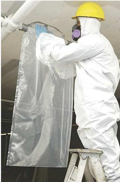
small scale removal jobs on pipes or other non-flat surfaces. The glovebag temporarily surrounds the pipe in a way that retains all released asbestos fibers within the bag. Tent procedures can be used only for removal of less than 260 linear feet or 160 square feet of ACM.
