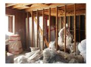
tape. Remove with minimum possible disturbance – score (make a shallow cut) with a utility knife; use a crowbar instead of a hammer. Remove at least 6 inches to 2 feet beyond visible mold growth or water stains on front and back sides. Double bag for safe disposal.
